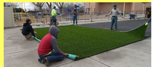
Synlawn installing the preschool playground turf.
